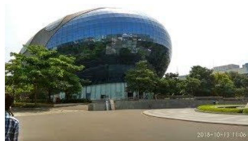
Figure 3.1.2 Massive curve structure with glass façade
