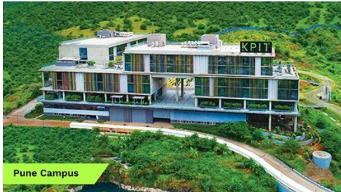
Figure 3.3.1 External Façade showcasing the fins on southern side
