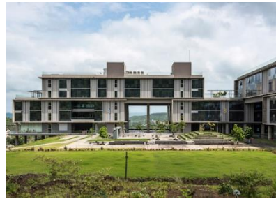
Figure 3.3.2 External façade of the office building
