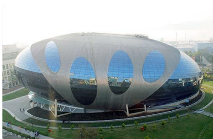
Figure 3.1.1 The curve is encircled with steel and Aluminum cladding
