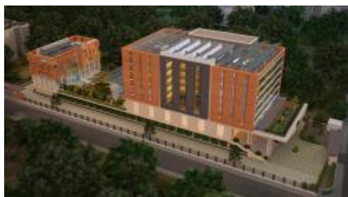
Figure 3.4.1 External façade of the office structure
